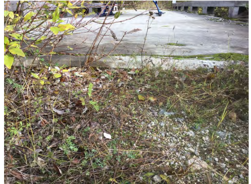
Deck elevation 100mm higher than road elevation
