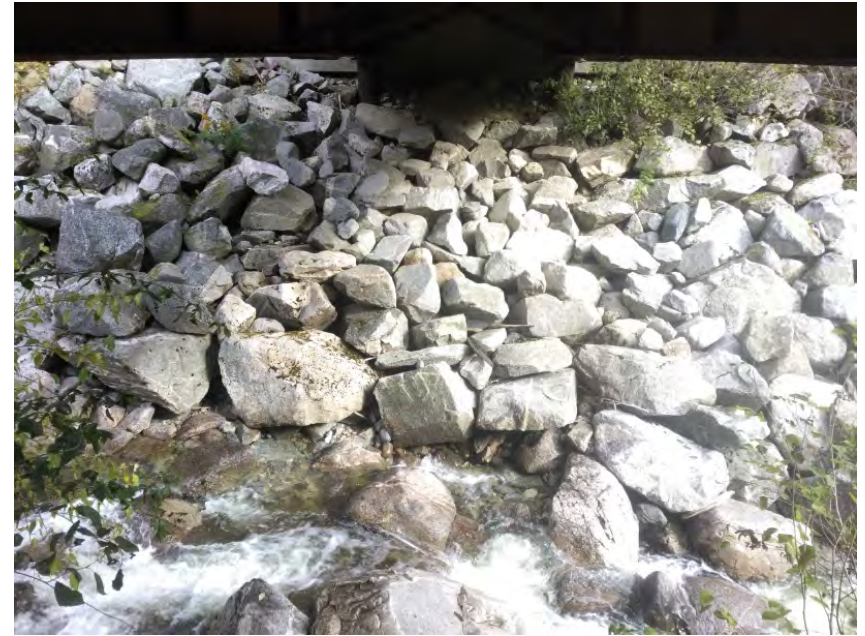
Left Bank Abutment when facing downstream
