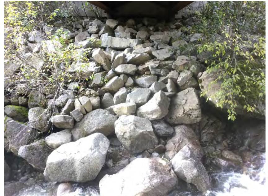
Right Bank Abutment when facing downstream
